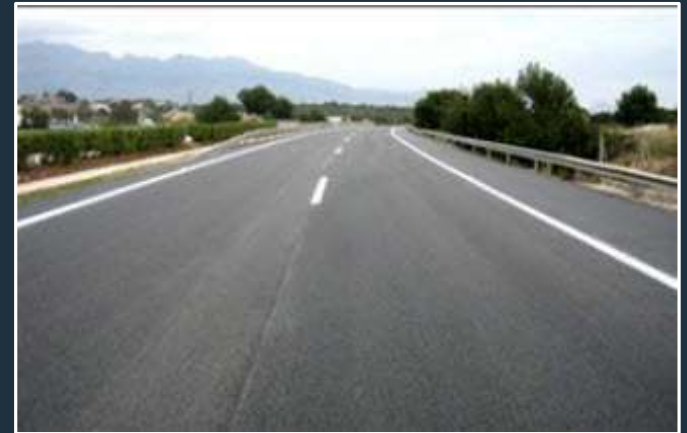
Rubberized asphalt pavement in service
