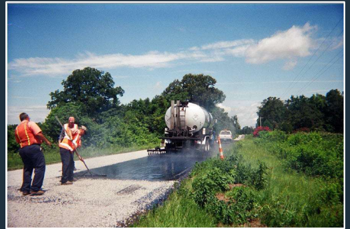
Spraying the asphalt-rubber membrane
