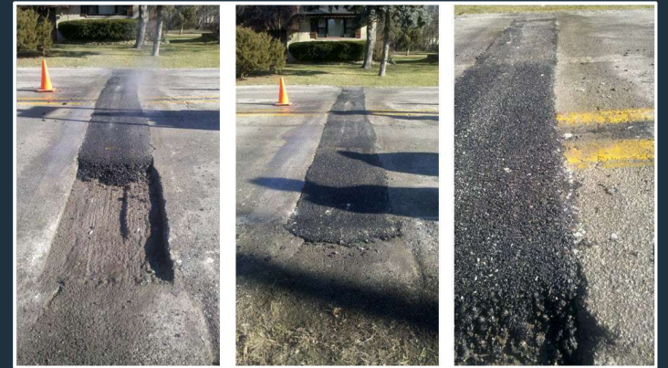
Rubberized patch placement
